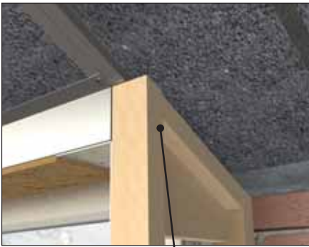
Infill 95 x 362mm In this case infill option is shown as timber. Intrusion panel is cut to accommodate the infill.
