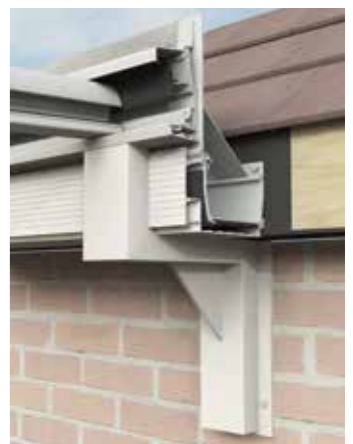
Custom designed gallows brackets are sometimes required
