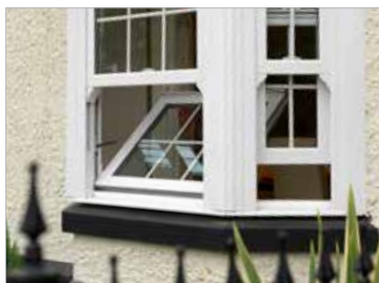
...and tilt inwards, for easy cleaning from within the building
